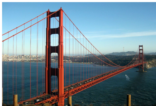
Figura 1.5 – Ponte Golden Gate
